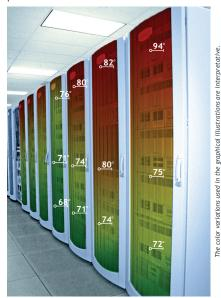
Before KoldLok products were installed, a foam product was used to plug holes and fans were used to cool the computer room. Temperatures reached 94°F, 17 degrees higher than is recommended by the American Society of Heating, Refrigerating, and Air-Conditioning Engineers (ASHRAF).
