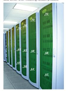
After KoldLok products were installed, virtually all temperatures dropped below the recommended 77°F, resulting in increased cooling optimization and greater overall data center efficiency.
